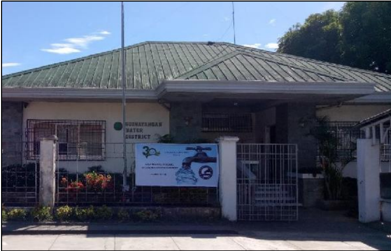
Figure 1. The Guinayangan Water District Main Office Provincial Road, Brgy. Calimpak, Guinayangan, Quezon Hotline # - (042) 717-6027 Smart # 09282443768
